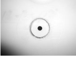
3. Insert an Allen wrench or screwdriver into the pilot hole from the hole saw to prevent the plug from falling into the tank. Then cut the rest of the way through the tank with a utility blade and remove the plug from the tank.
