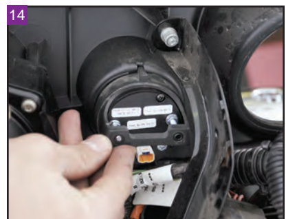
Reinstall the stock mounting bridge.
