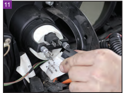
Disconnect the wiring from the battery, oil pressure, fuel and air temperature gauges.
